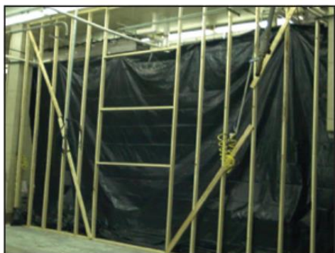
Temporary barriers can protect the production environment from aerosols and traffic that may carry Listeria exposed during construction.
